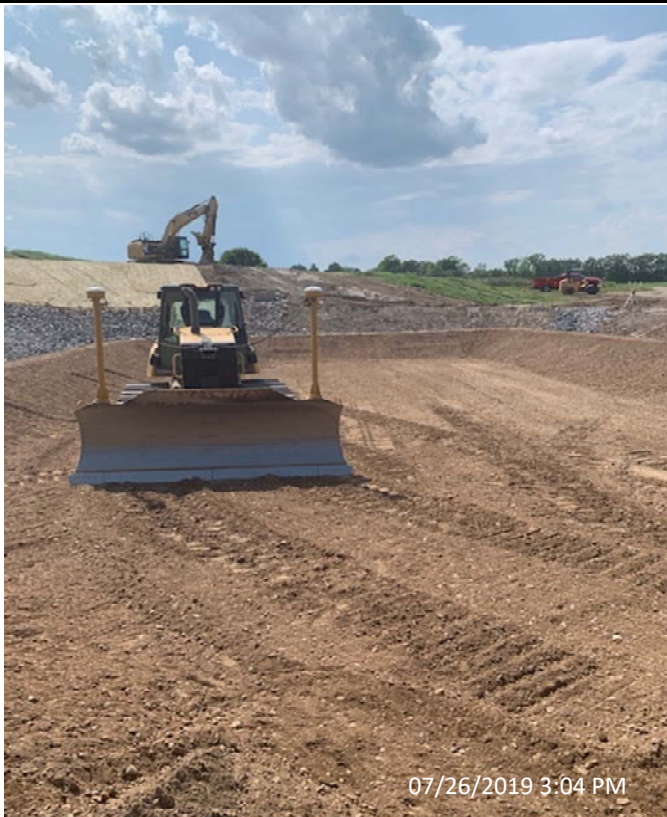
Photo 30- Grading LSTA Type 2 Stone
