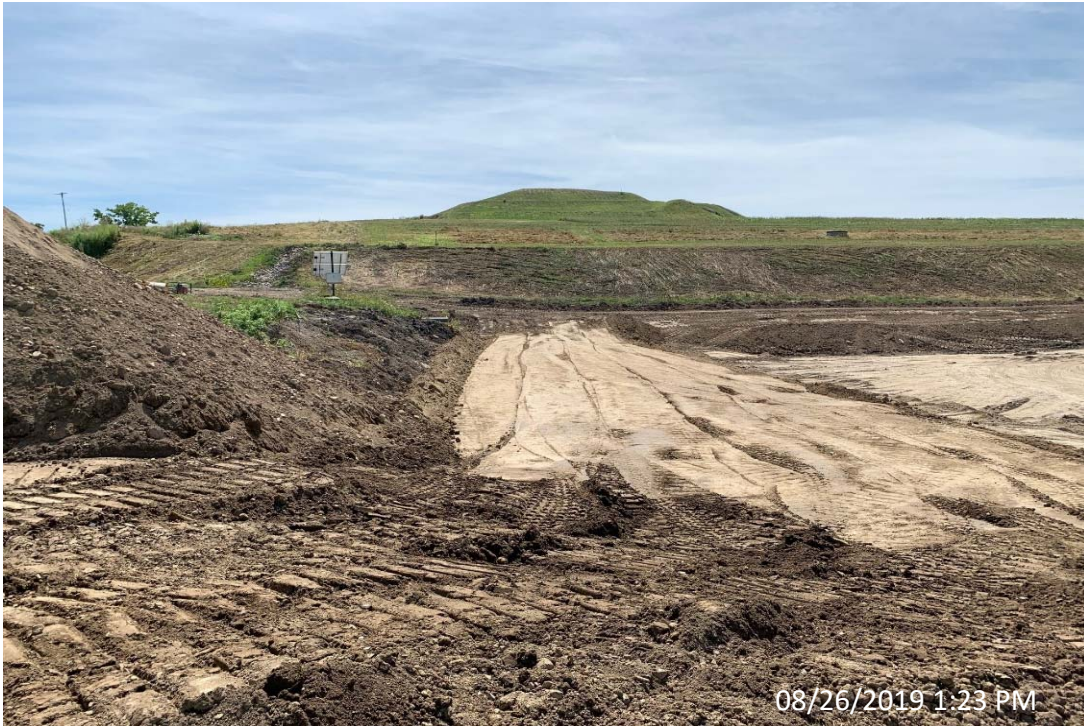
Photo 47- Settling Pond North Slope Filling Looking South
