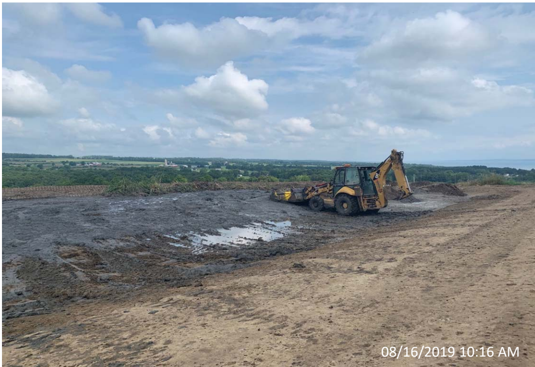
Photo 45- Sediment Disposal in Confined Disposal Area Looking Northwest
