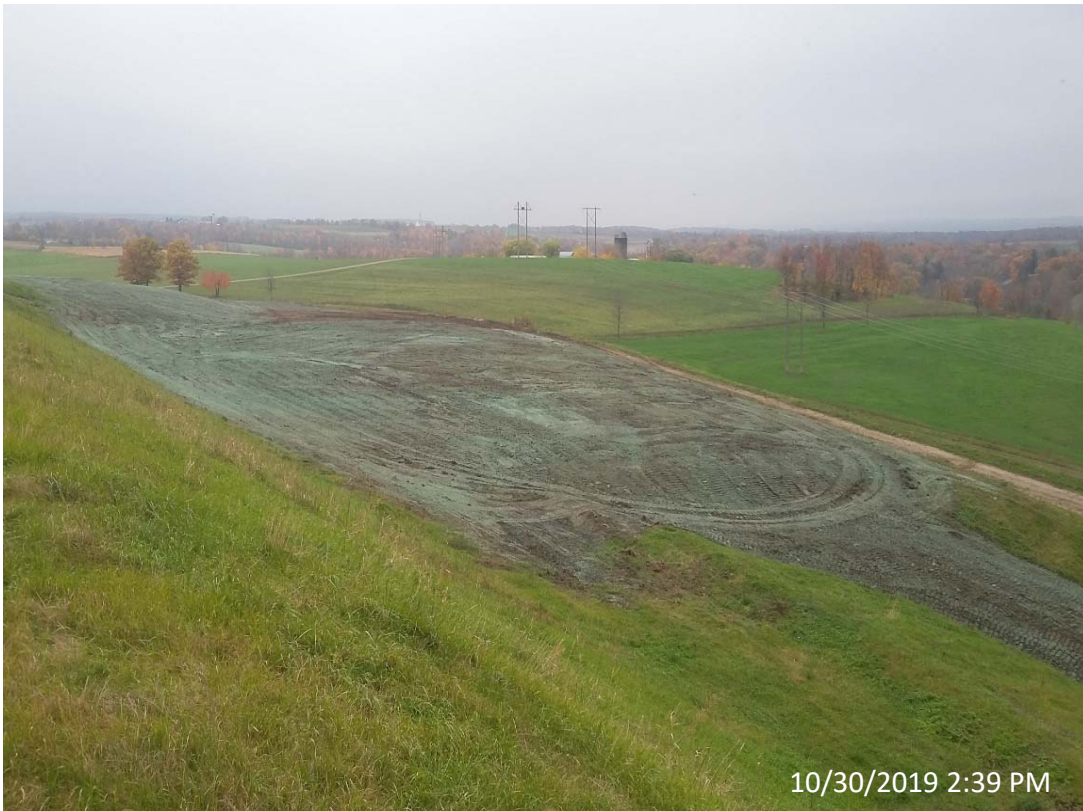
Photo 68- Graded, Covered, and Hydroseeded Sediment Disposal Area
