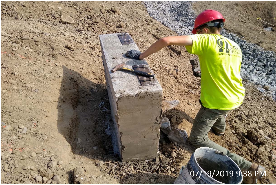
Photo 13- LSTA Pipe Bridge Concrete Footer
