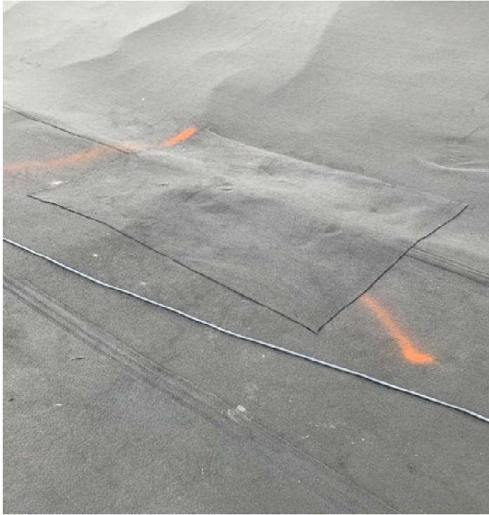
Photo 27- Cushion Geotextile Repair
