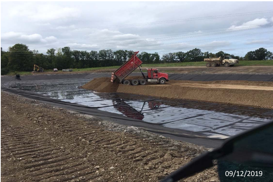
Photo 59- Settling Pond Type 2 Stone Placement Looking Northwest
