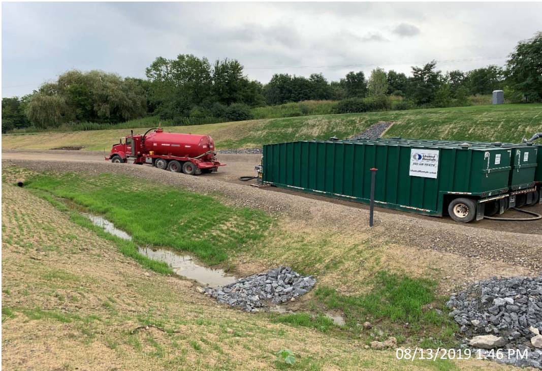
Photo 41- Vacuum Truck in LSTA Looking Southeast
