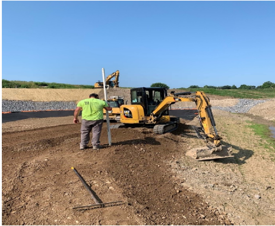
Photo 31- Checking LSTA Type 2 Stone Thickness
