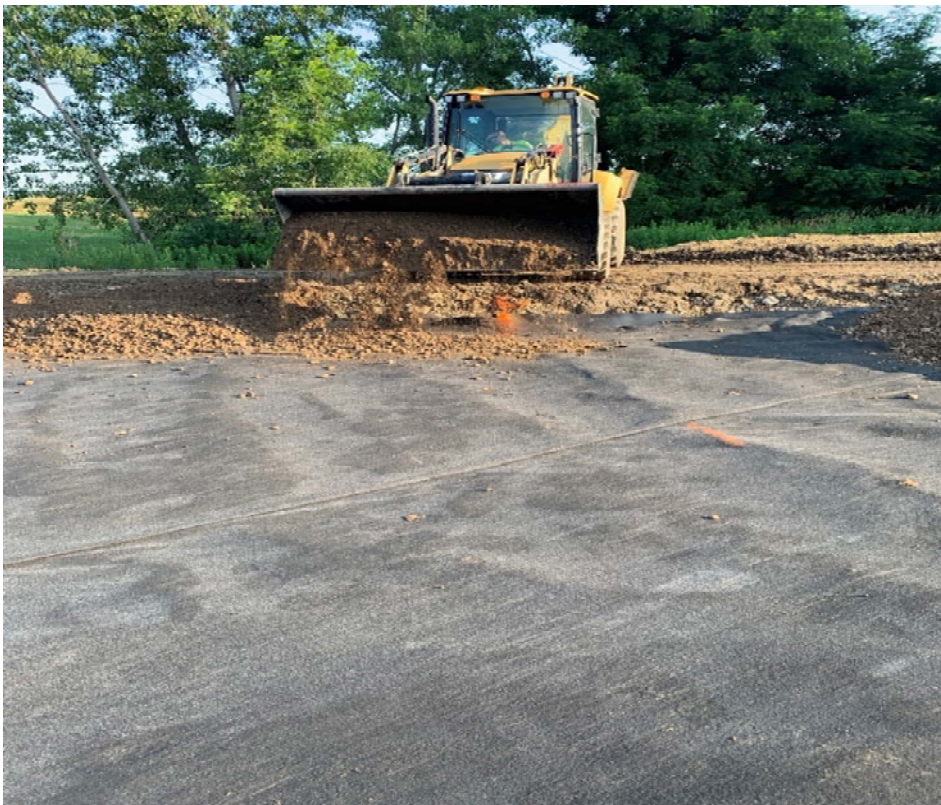
Photo 28 - Type 2 Stone Placement Over Cushion Geotextile
