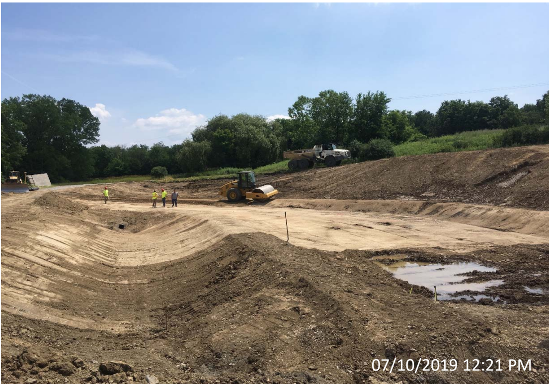
Photo 8 - LSTA Subgrade Preparation Looking East
