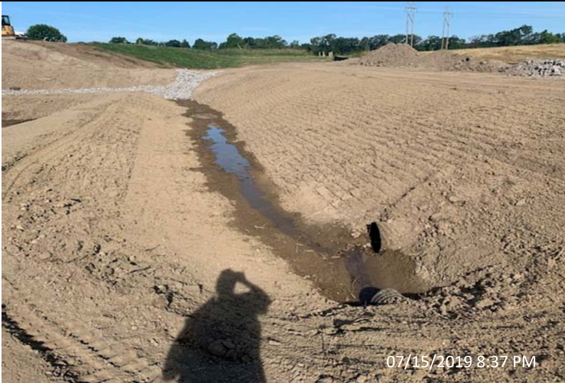
Photo 10- North Drainage Channel at Culverts Looking West
