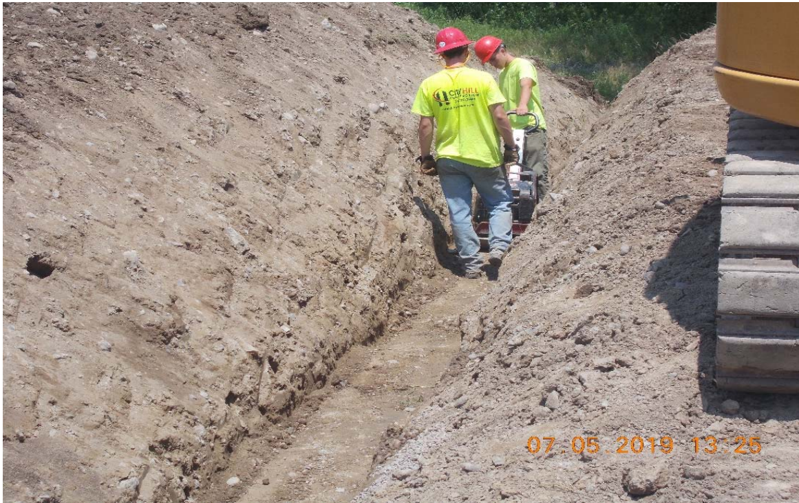
Photo 3- LSTA Porewater Discharge Pipe Trench Compaction
