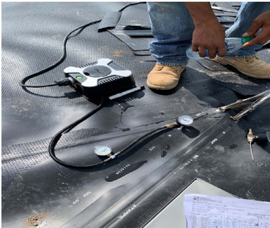
Photo 24- Geomembrane Non-Destructive Seam Air Pressure Testing
