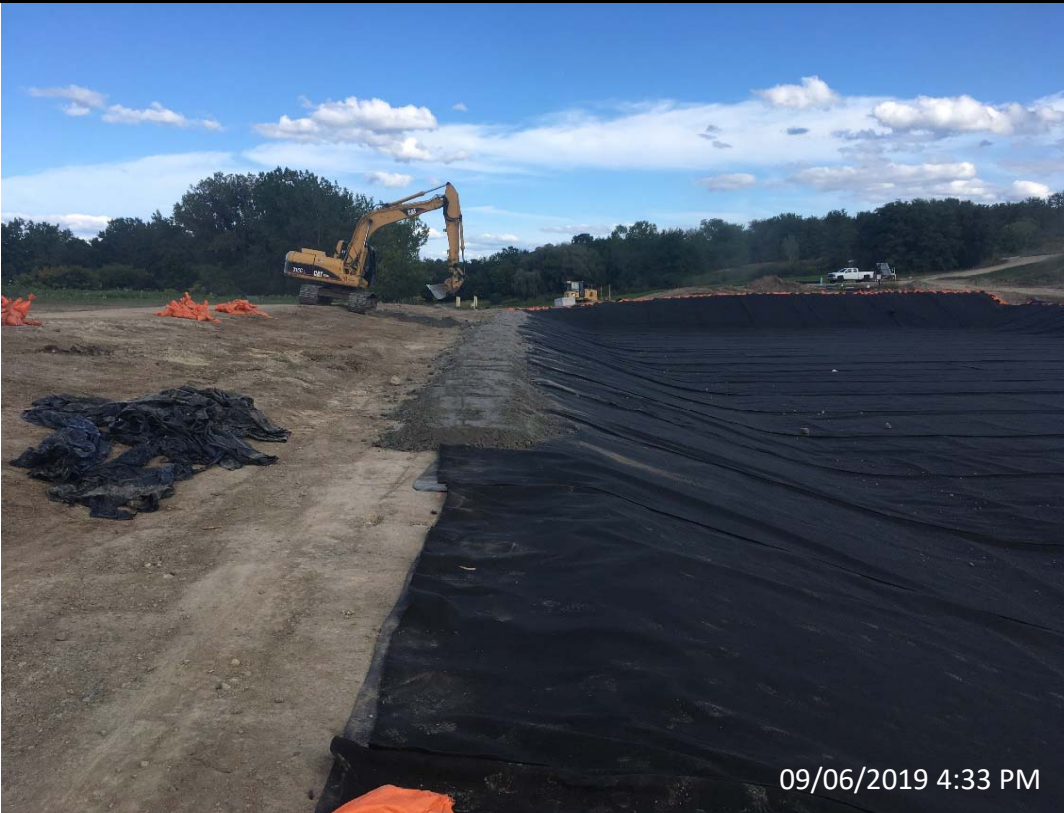
Photo 56- Low Permeability Backfill Placement Over Settling Pond Runout Looking East
