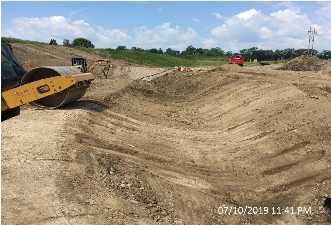
Photo 9- Compacting North Berm Looking West
