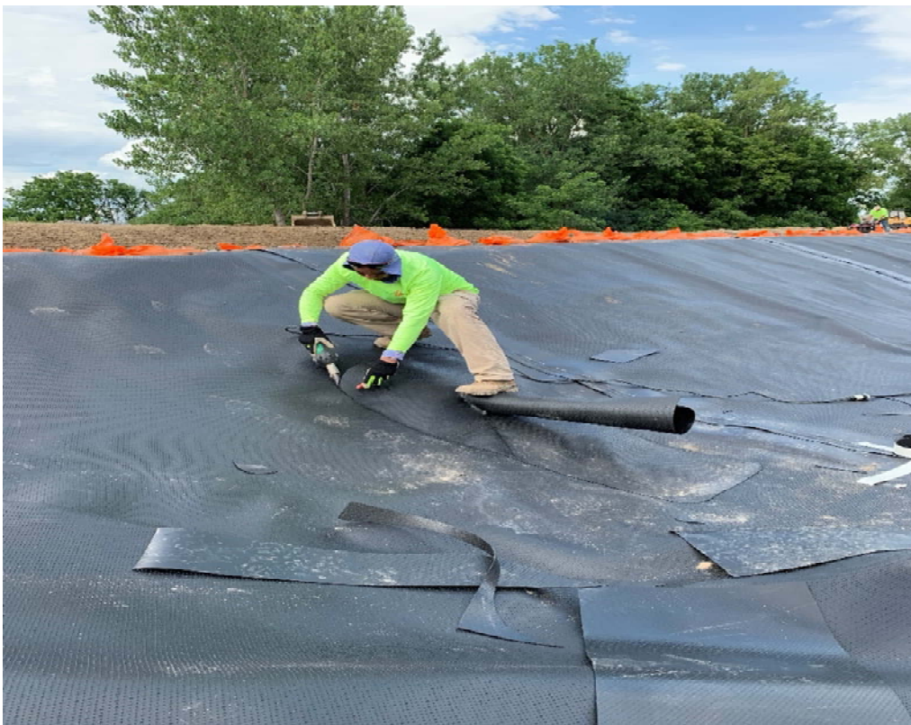
Photo 22- Geomembrane Boot Installation at LSTA Discharge Pipe
