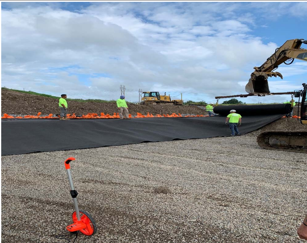
Photo 16 - LSTA Porewater Geocomposite Placement over No. 1 Stone Subgrade
