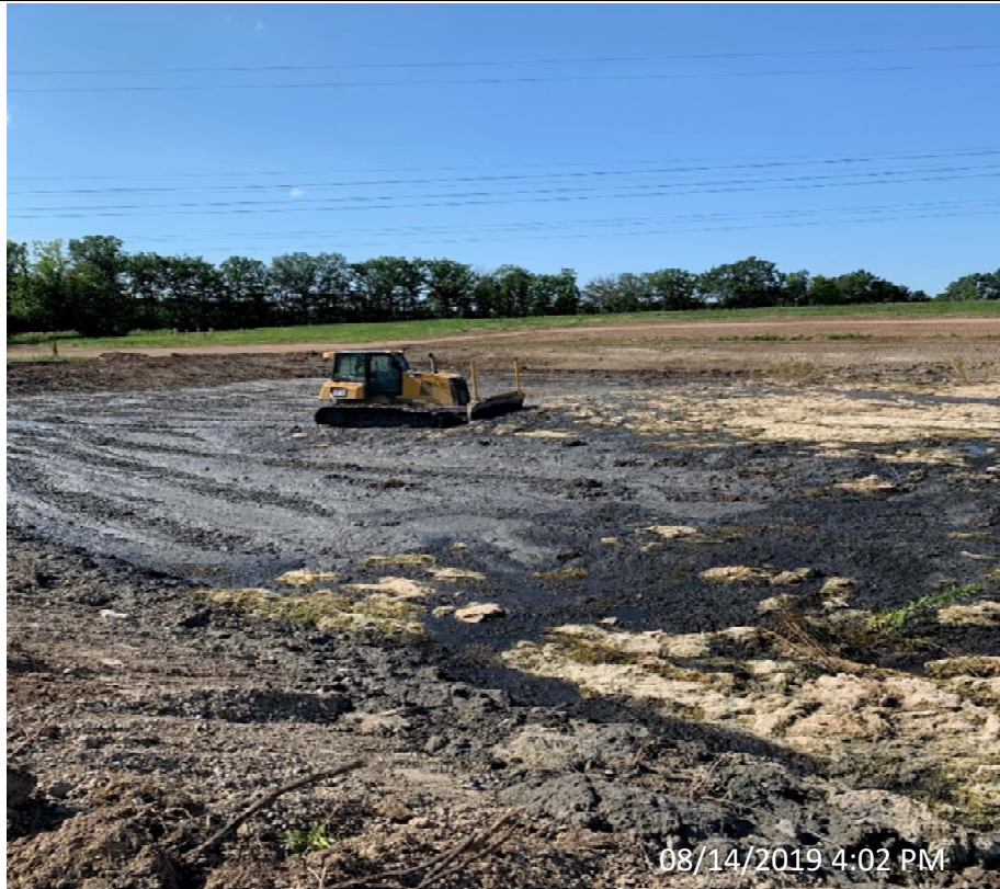
Photo 44- Bulldozing Settling Pond Sediment to the East Looking Northwest
