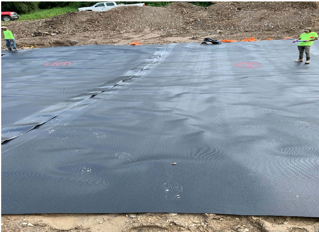
Photo 20 - LSTA 60-mil HDPE Geomembrane Installation
