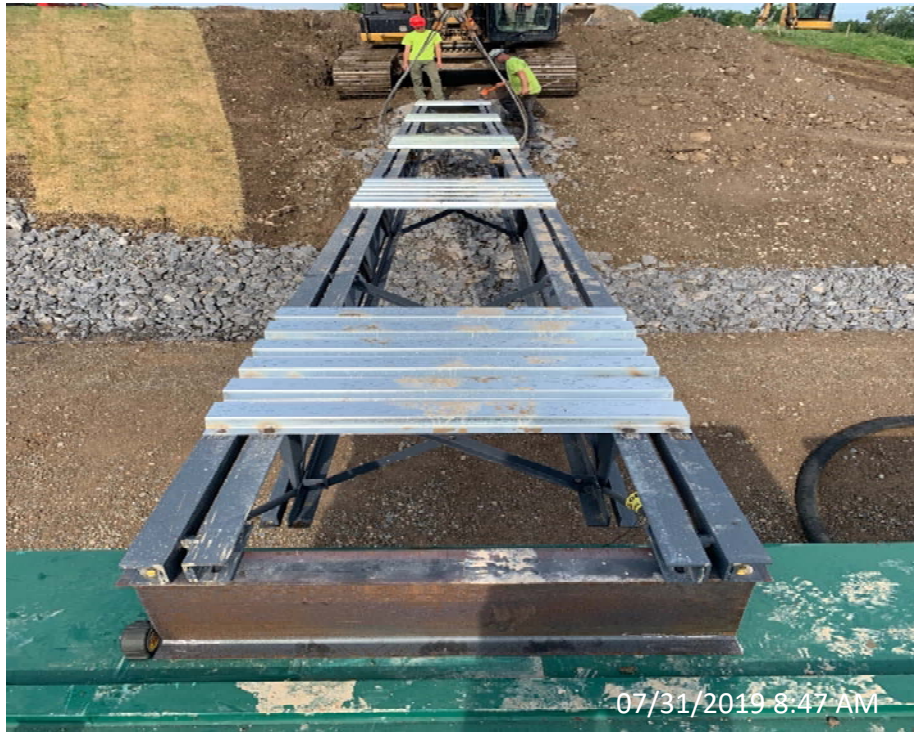
Photo 37- Placement of LSTA Pipe Bridge Looking West
