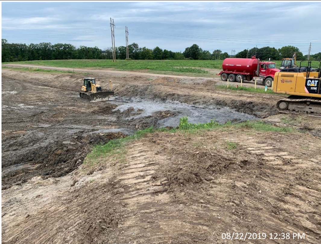
Photo 46- Settling Pond Sediment Removal From Northeast Corner
