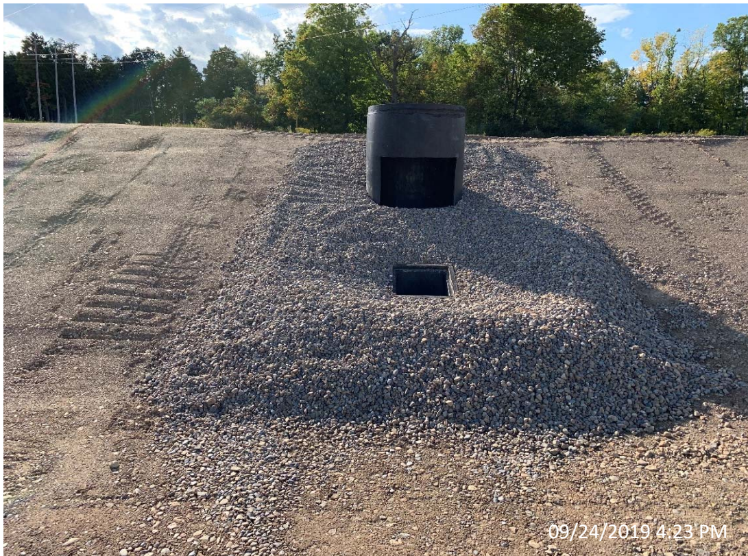
Photo 64- No. 2 Stone Placement Around Settling Pond HDPE Outlet Structures
