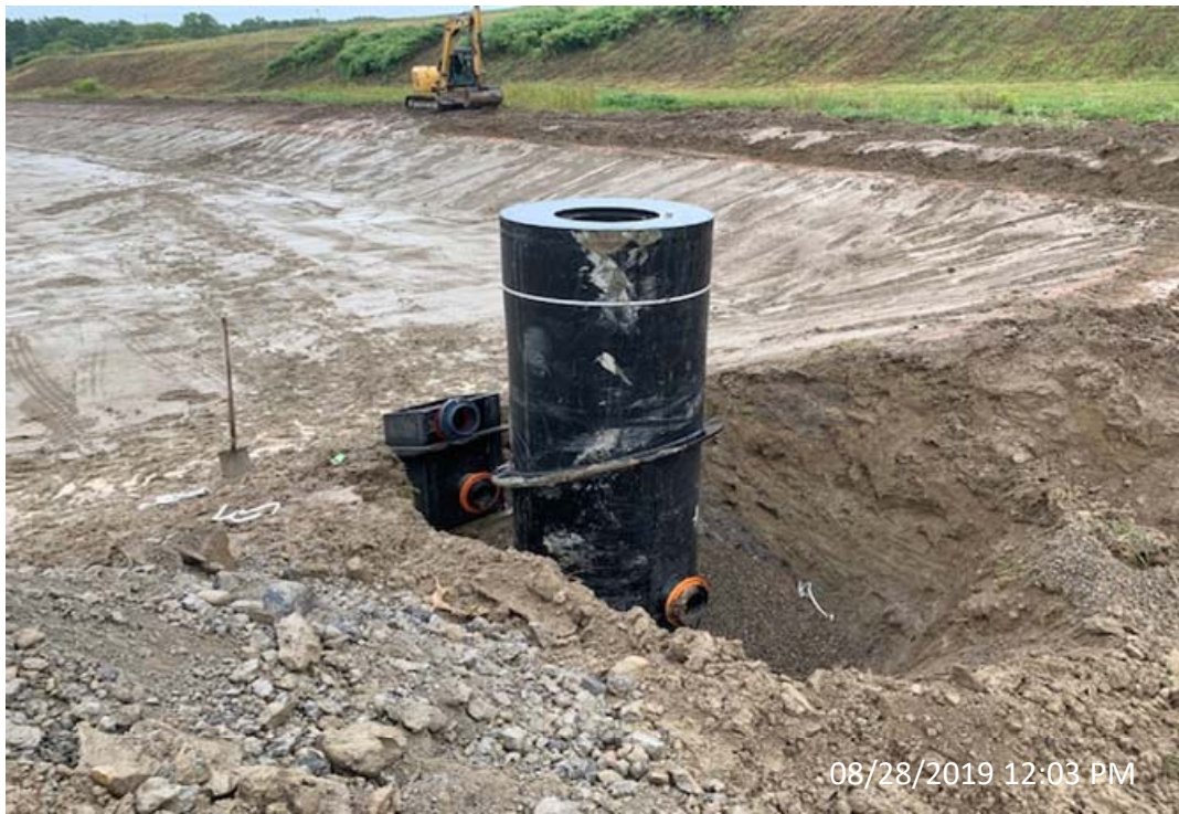
Photo 49- Settling Pond HDPE Outlet Structures Installation
