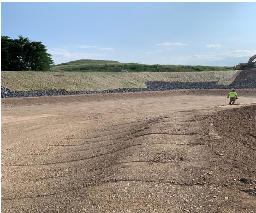
Photo 34 - LSTA Compacted Type 2 Stone Looking Southwest
