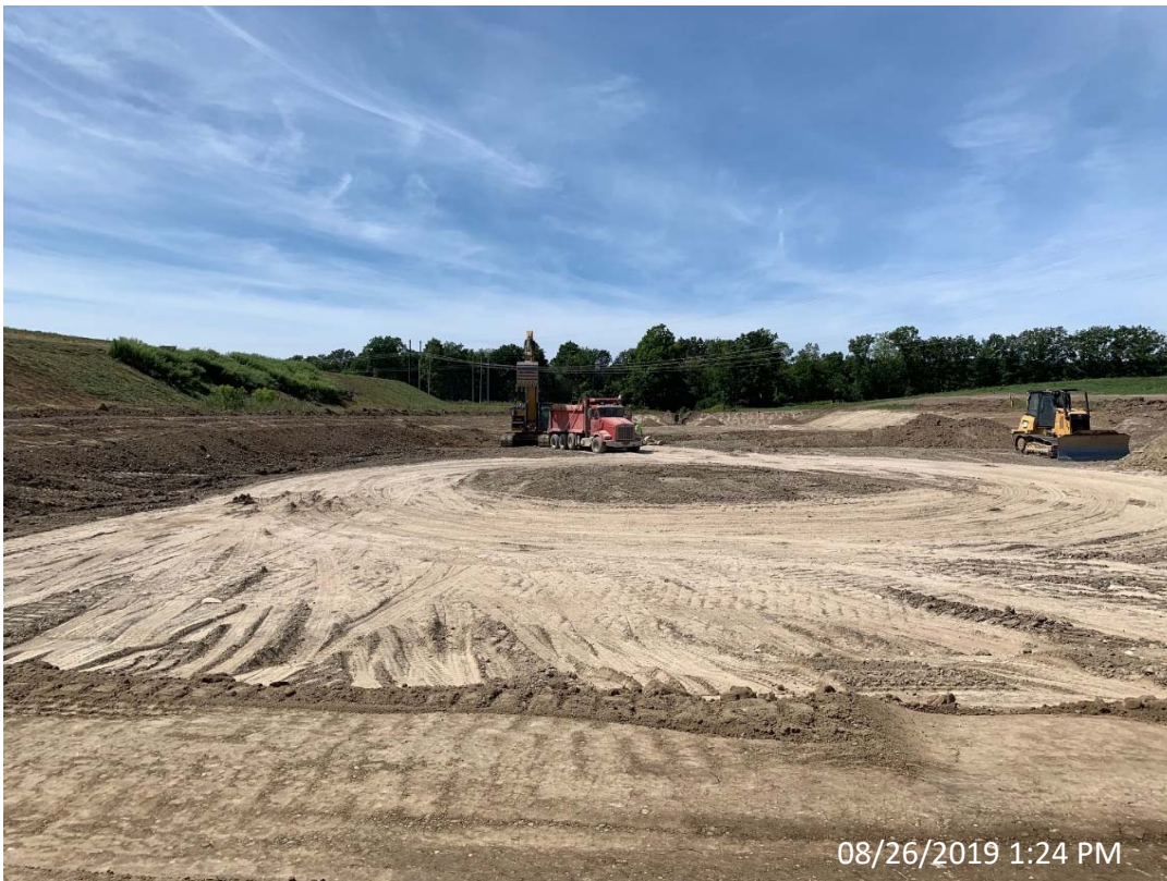
Photo 48- Excavation to Settling Pond Subgrade
