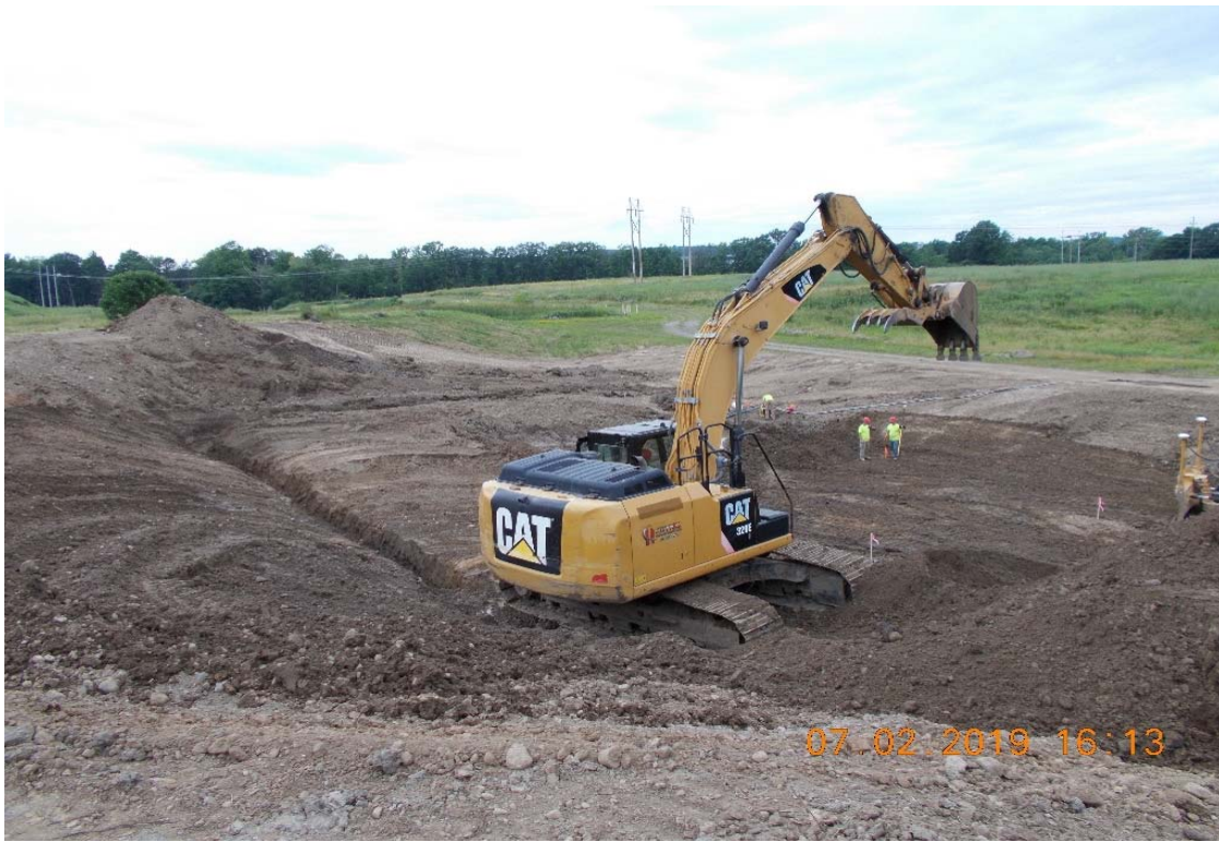
Photo 1 - LSTA Subgrade Excavation Looking Northwest
