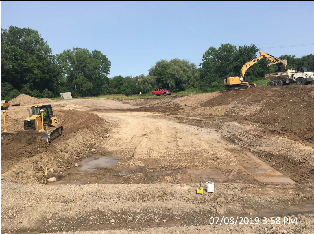
Photo 6- Nuclear Densometer Testing on the West Berm Looking East
