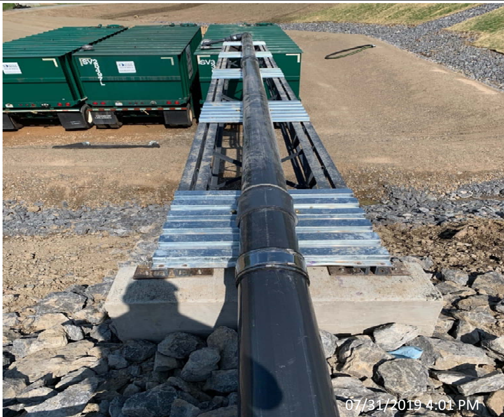
Photo 38- LSTA Pipe Brige Pipe Installation Looking East
