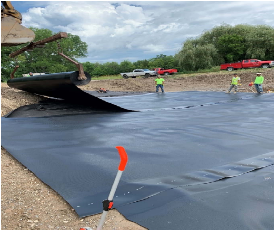
Photo 19- LSTA 60-mil HDPE Geomembrane Placement
