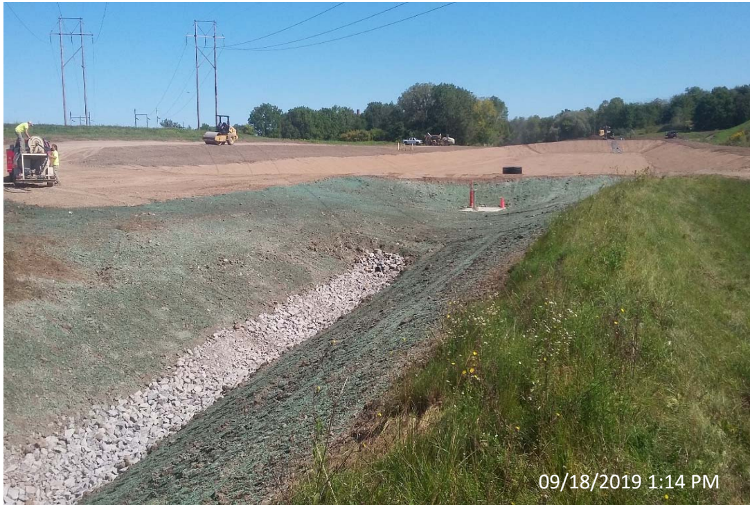
Photo 63- Settling Pond Discharge Channel Looking East
