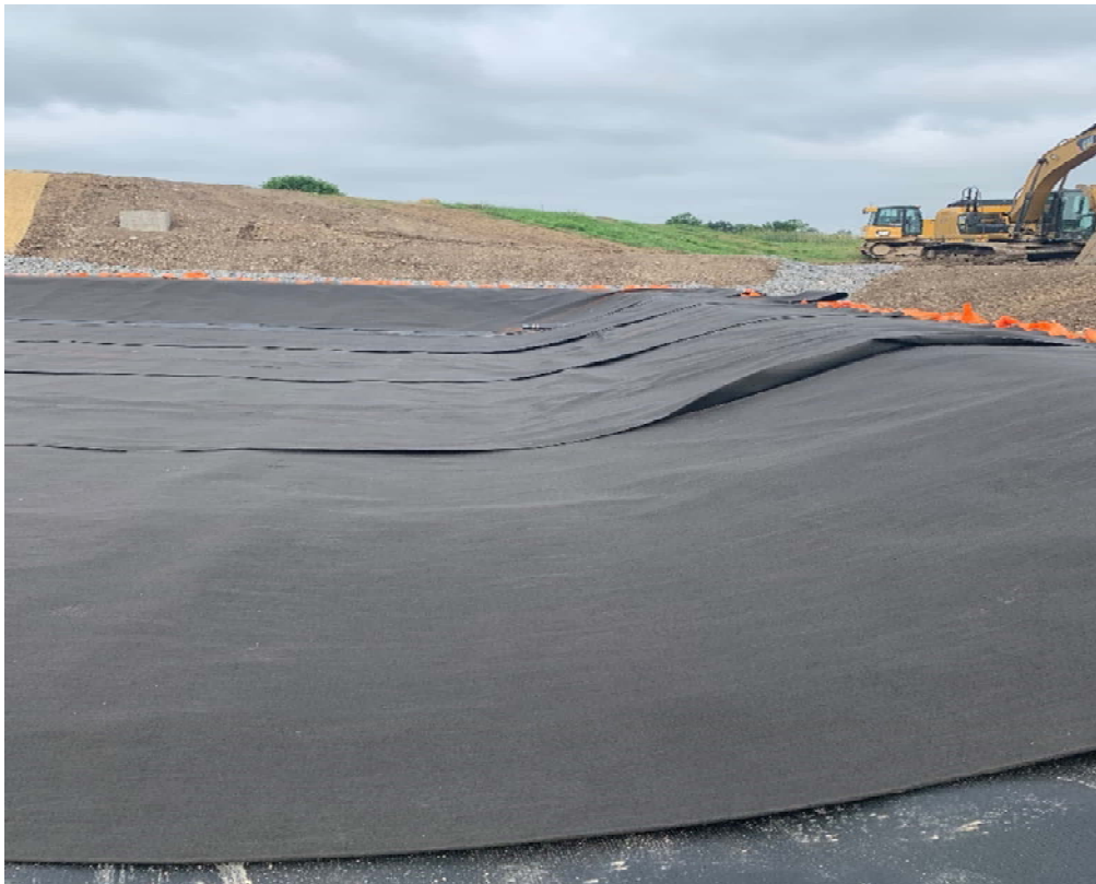
Photo 26- LSTA Cushion Geotextile Placement
