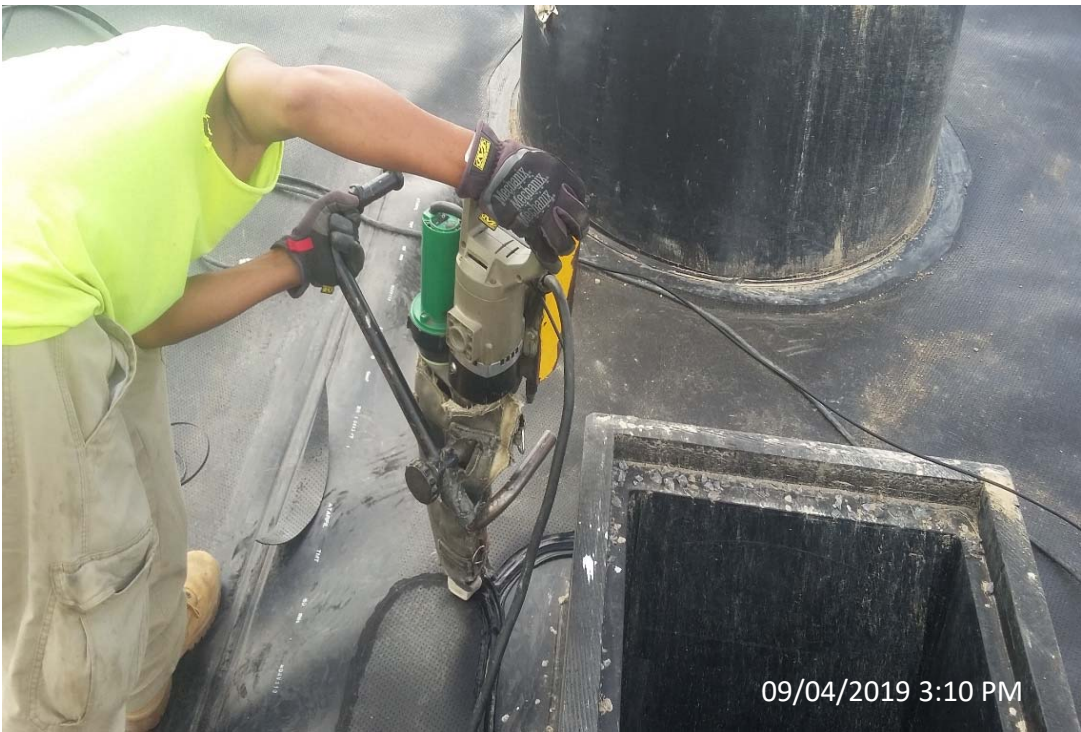
Photo 51- Extrusion Welding Geomembrane to HDPE Outlet Structure Skirt
