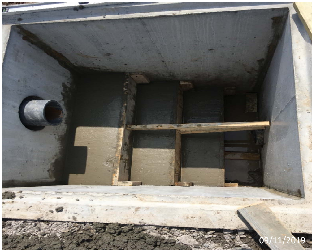
Photo 58- Settling Pond Cascade Aerator Concrete Steps Installation
