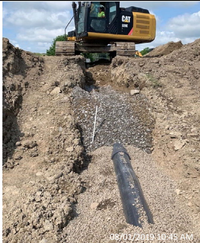
Photo 40- Leachate Sewer Pipe Installation
