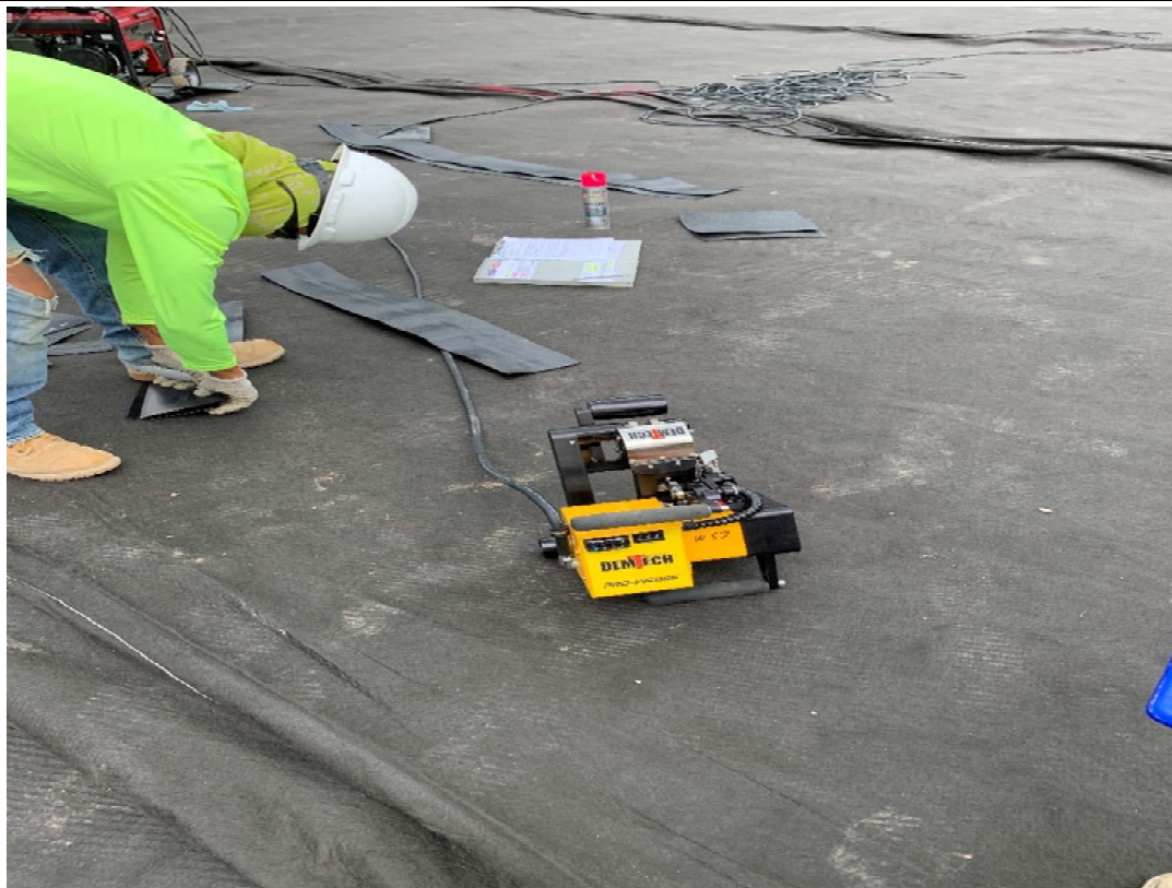
Photo 18 - LSTA Trial Weld Preparation
