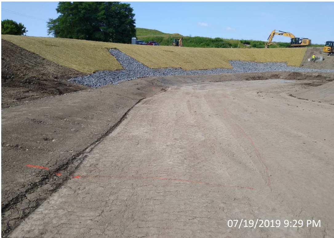
Photo 12- LSTA Subgrade Looking Southwest
