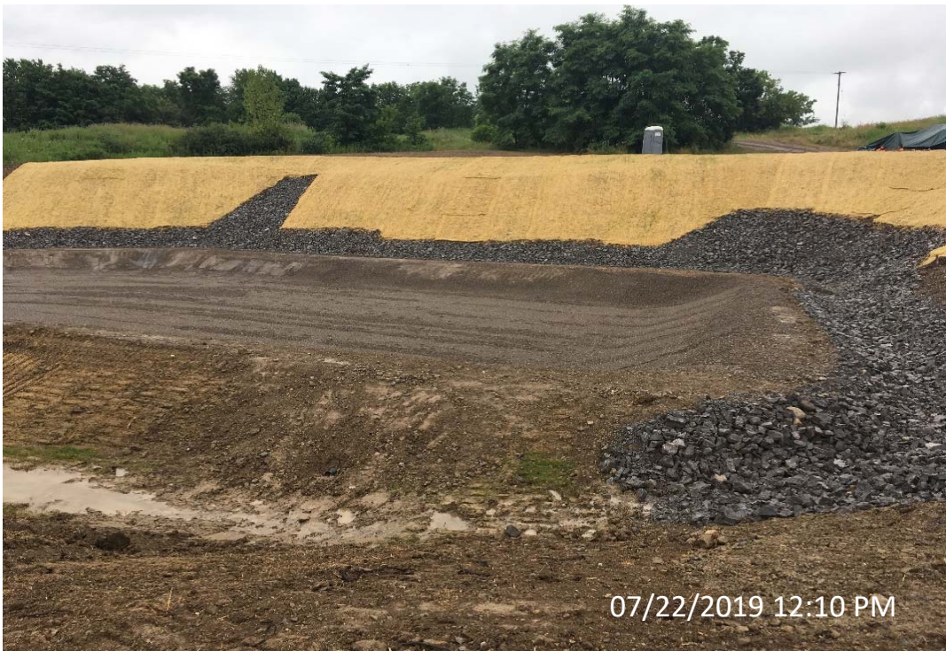
Photo 15- LSTA No. 1 Stone Subgrade Looking South
