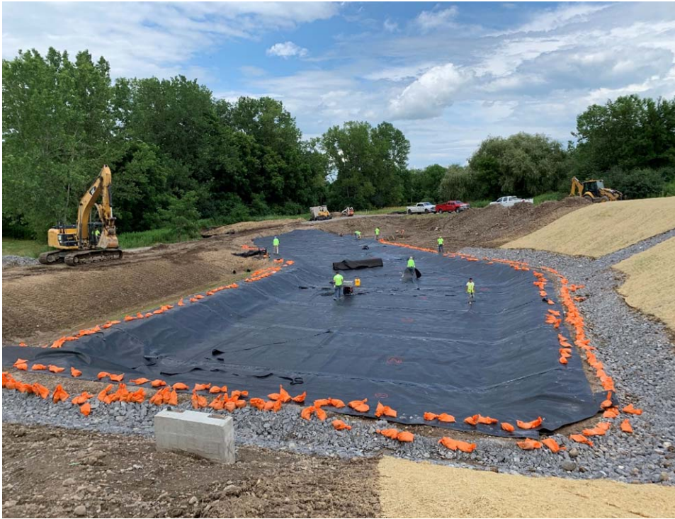
Photo 21- LSTA 60-mil HDPE Geomembrane Installation Looking East
