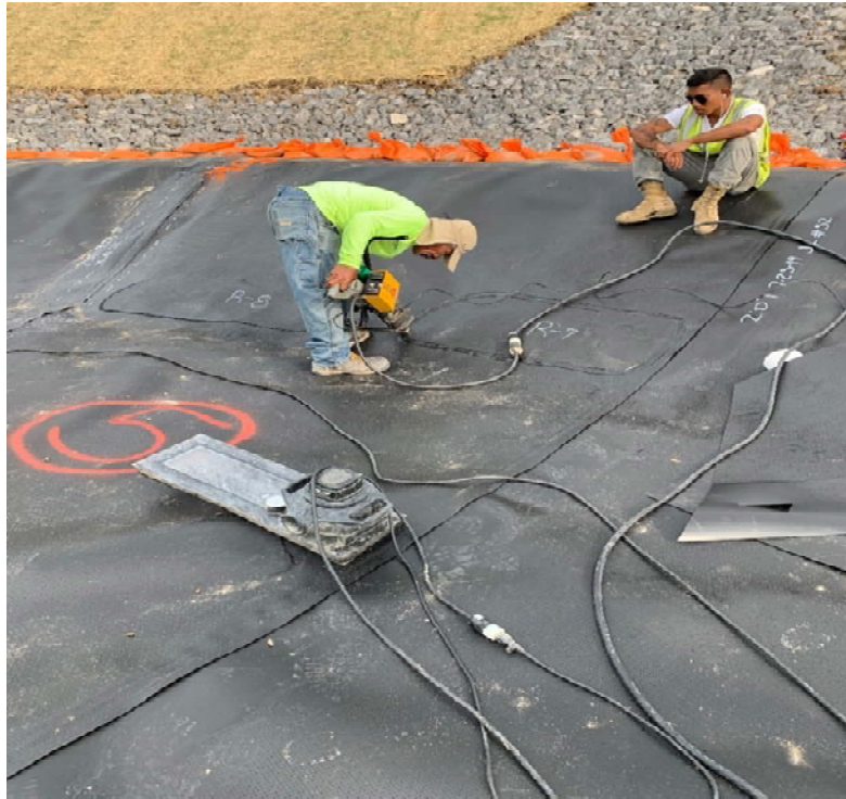
Photo 25- Geomembrane Repair Extrusion Welding and Vacuum Box
