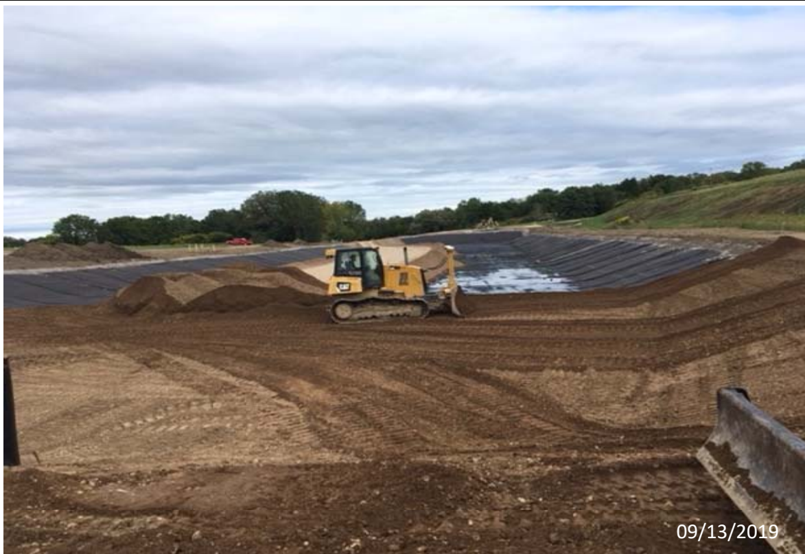
Photo 60- Settling Pond Type 2 Stone Grading Looking East
