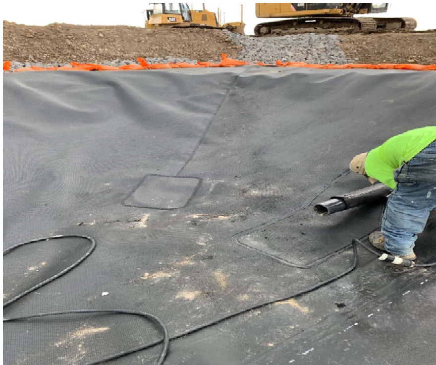
Photo 23- Geomembrane Boot Installation at LSTA Discharge Pipe
