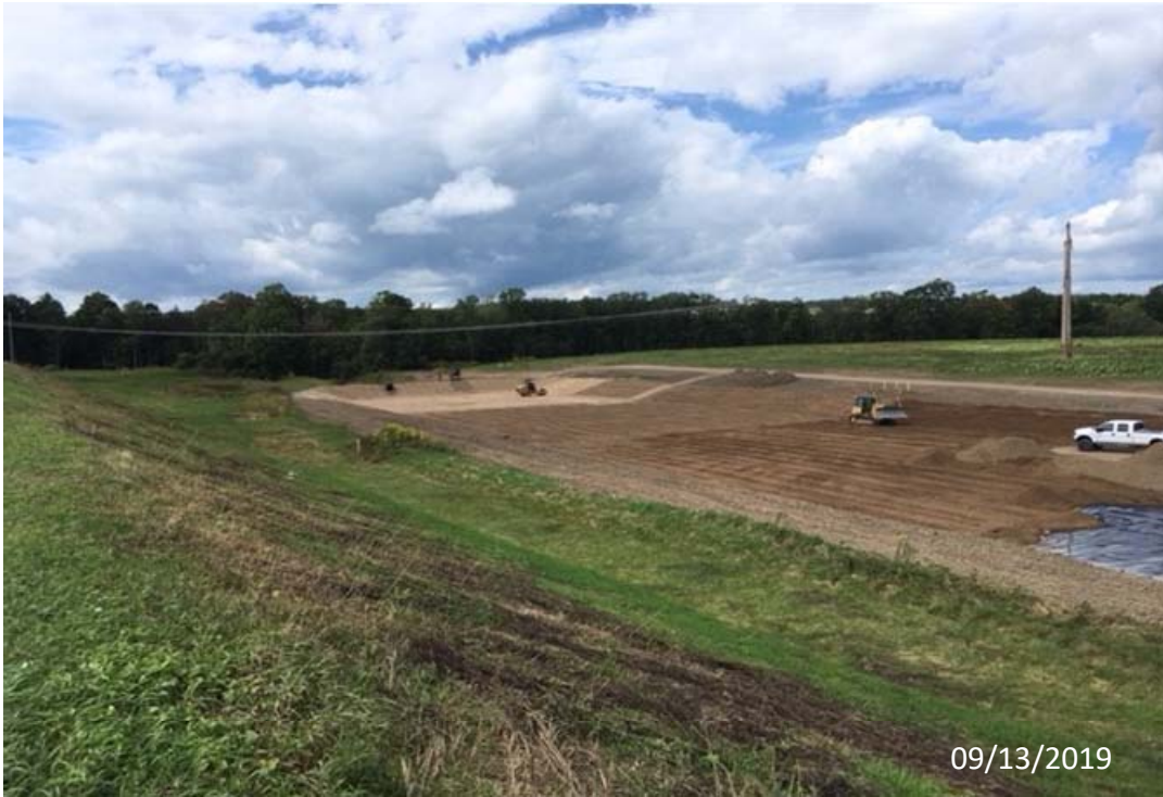
Photo 61- Settling Pond Type 2 Stone Placement and Compaction Looking Northwest
