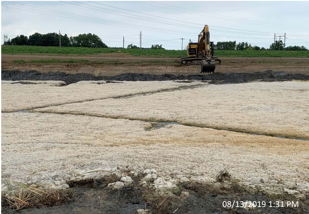
Photo 43- Excavating Trenches in Settling Pond Sediment Looking North
