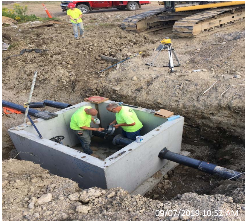
Photo 57- Settling Pond Outlet Gate Valve and Concrete Vault Installation
