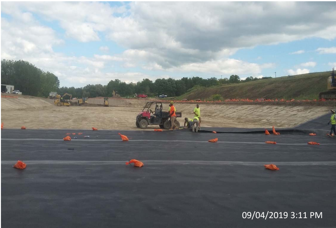
Photo 53- Settling Pond Geomembrane Deployment Looking East
