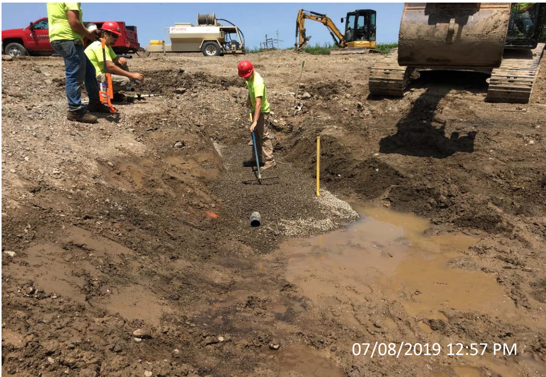
Photo 5- Porewater Discharge Pipe Installation Looking North
