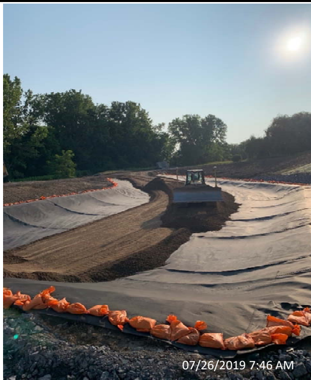
Photo 29- Placement of Type 2 Stone on the LSTA over the Cushion Geotextile
