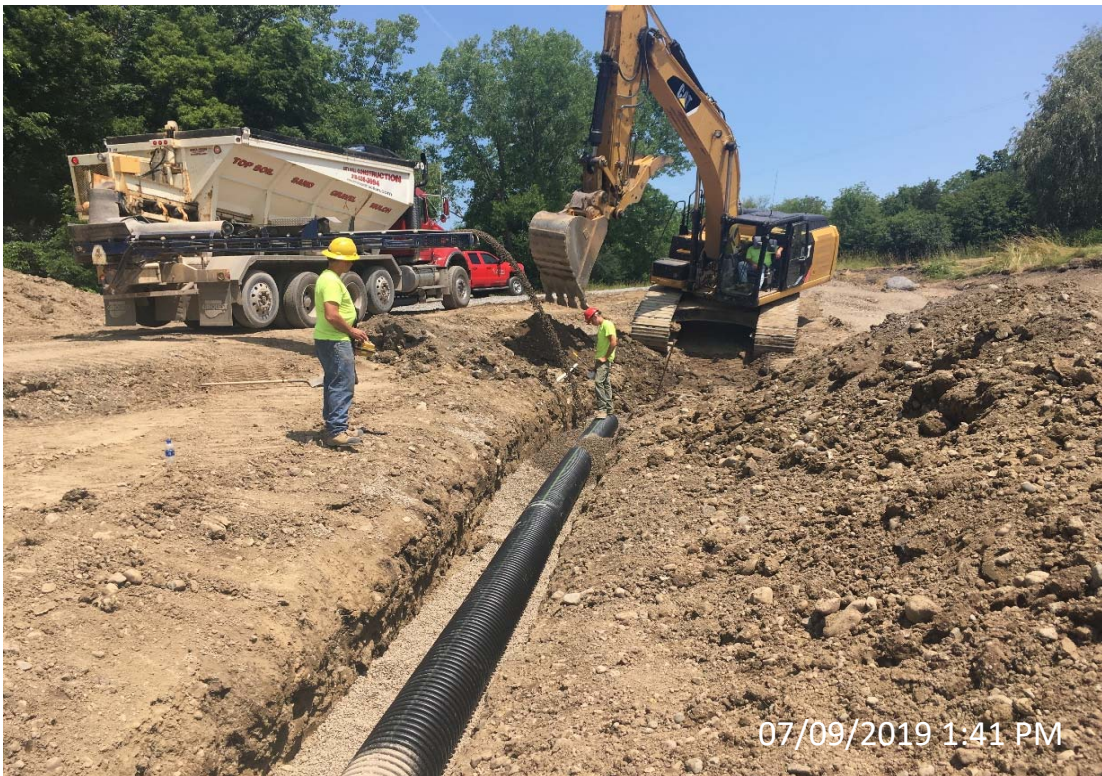
Photo 7- Northern 12- inch Culvert Installation Looking East
