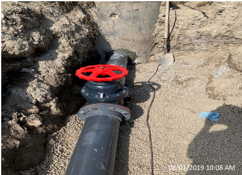
Photo 39- Gate Valve Installation at Manhole MH Common-1
