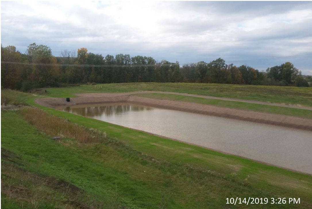
Photo 69- Finished Settling Pond Looking West
