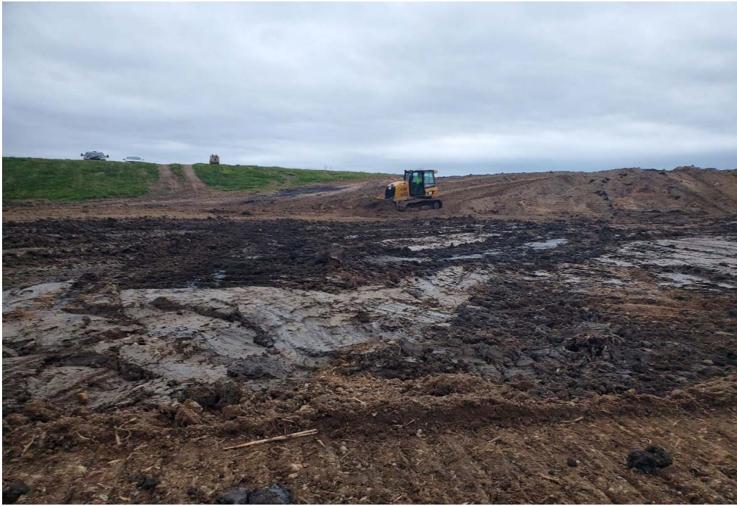
Photo 67- Sediment Stabilization and Grading Within the Confined Disposal Area
