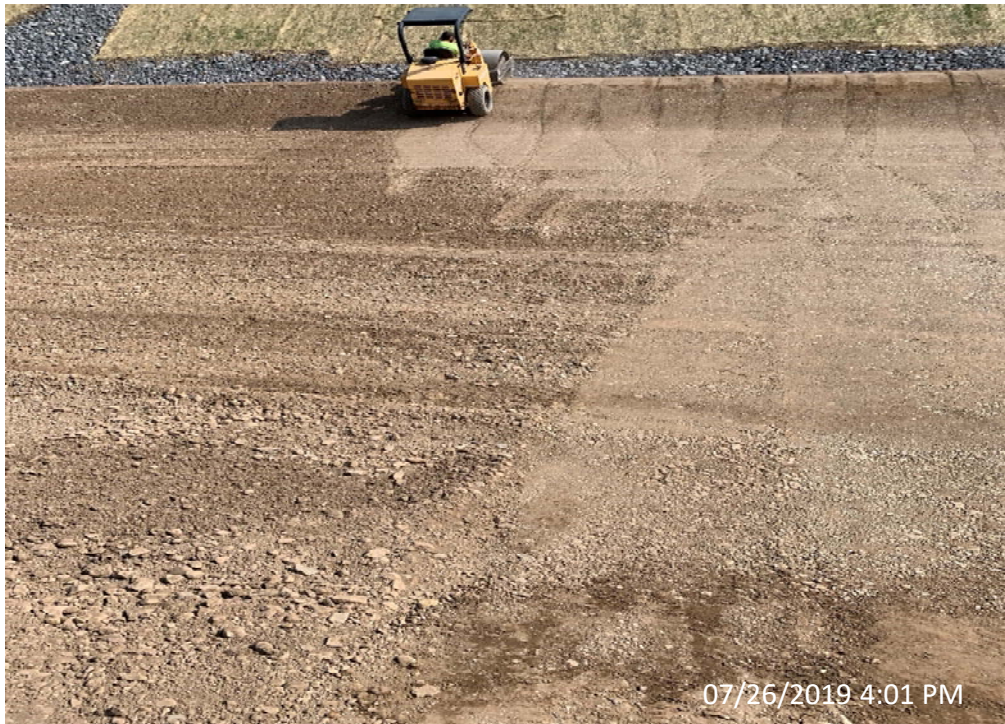
Photo 33- Compaction of LSTA Type 2 Stone Looking South
