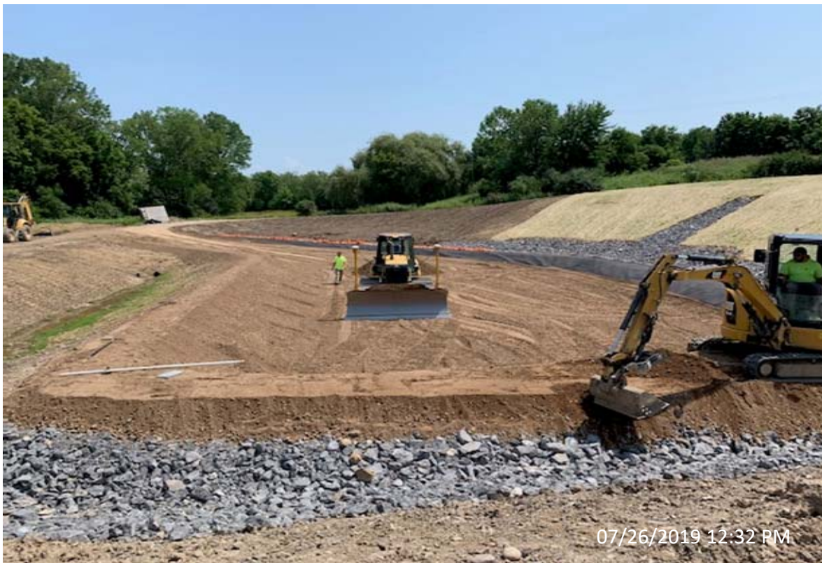
Photo 32- Grading LSTA Type 2 Stone
