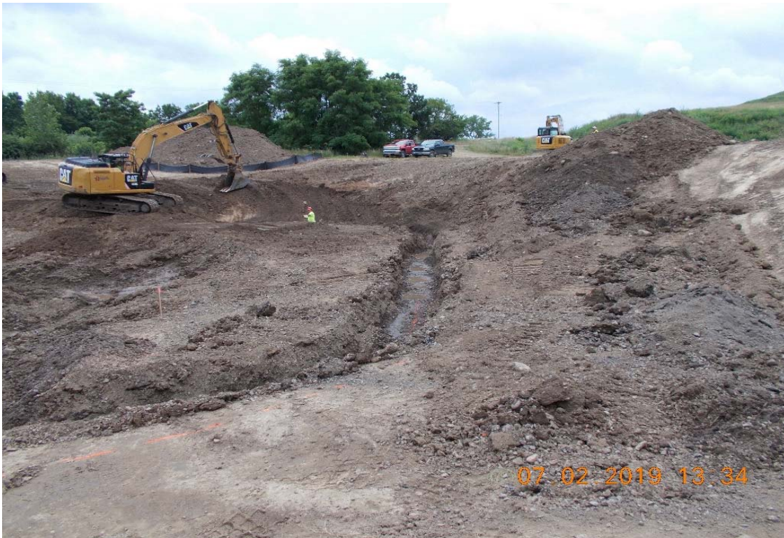
Photo 2 - LSTA Subgrade Excavation Looking East
