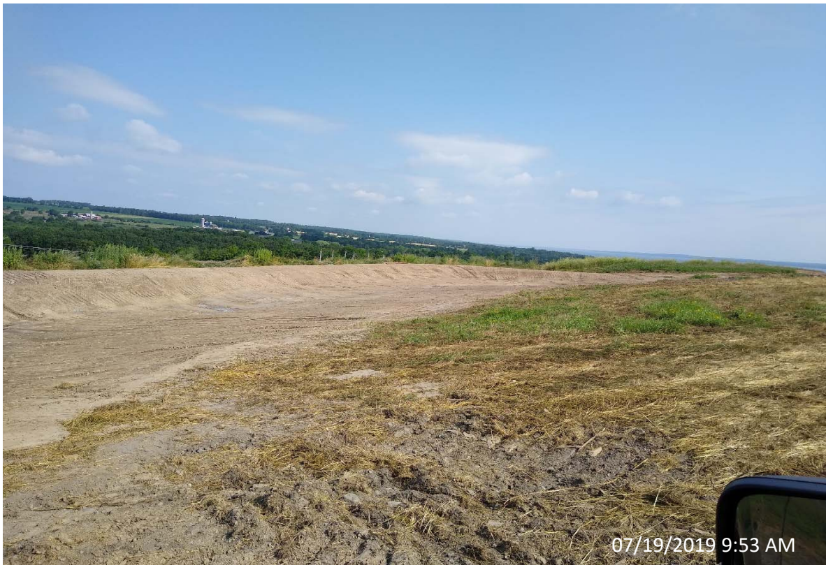
Photo 42- Confined Disposal Area for Sediment Disposal Looking Northwest
