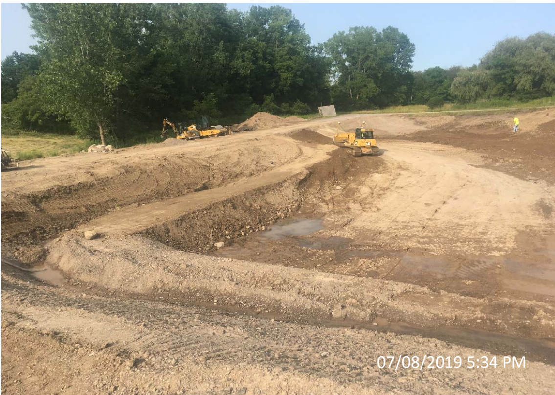
Photo 4- LSTA North and West Berm Construction Looking East
