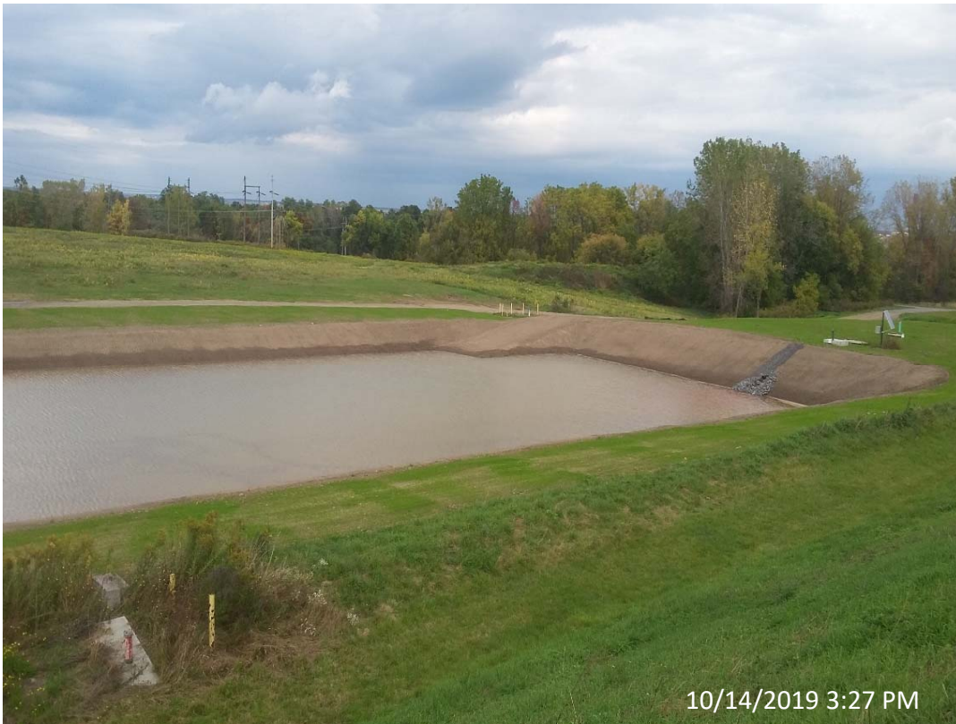
Photo 70- Finished Settling Pond Looking East
