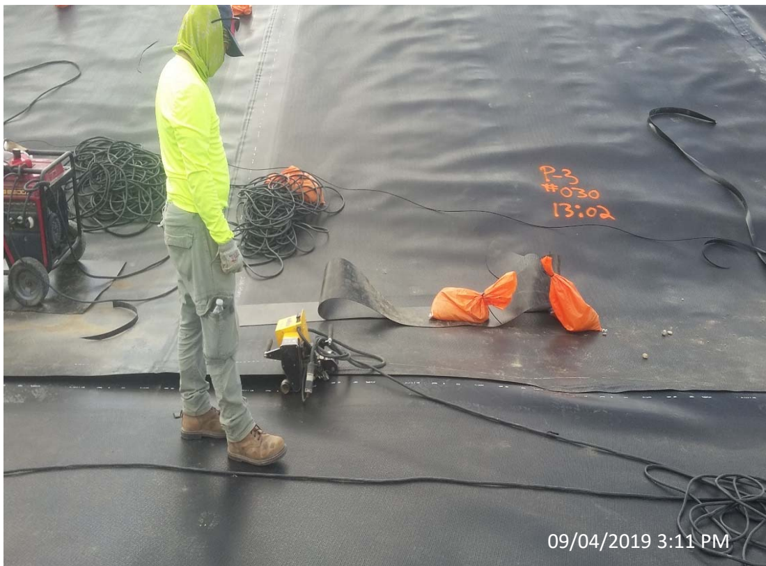
Photo 52- Fusion Wedge Welding Settling Pond Geomembrane
