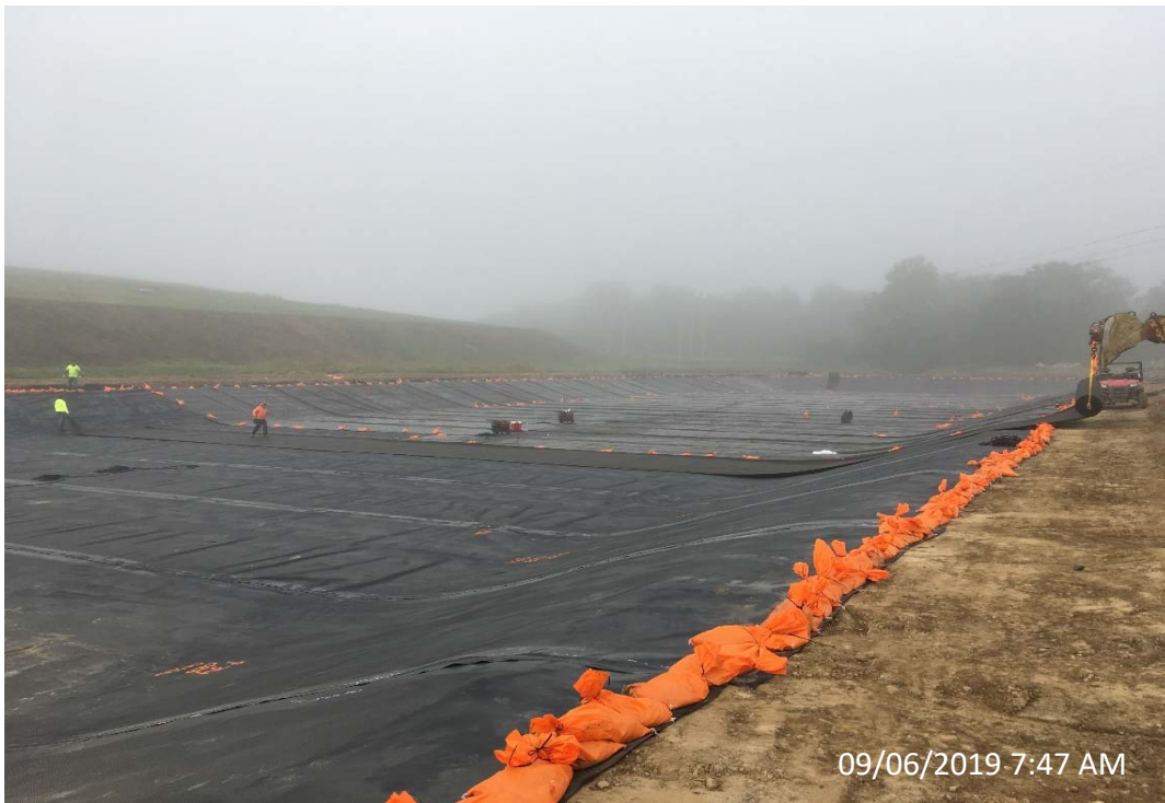
Photo 55- Settling Pond Cushion Geotextile Deployment Looking Southwest
