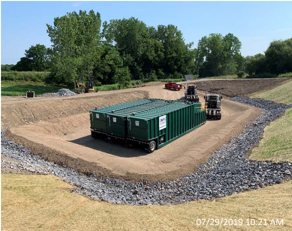
Photo 35- LSTA Storage Tank Placement
